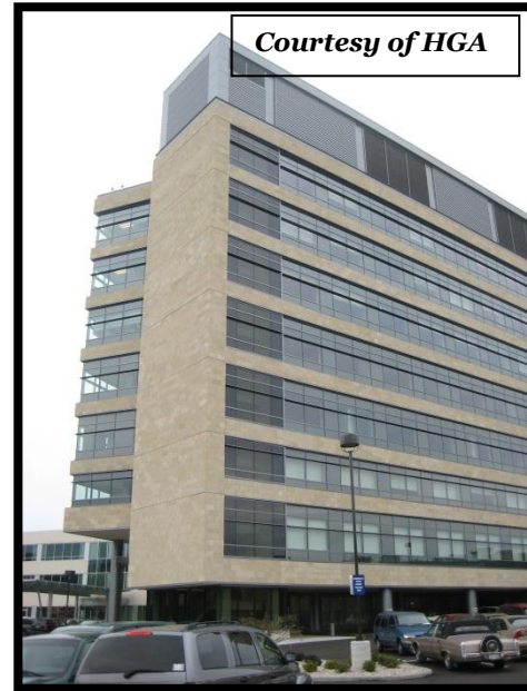
Picture 3: Bed Tower Addition
